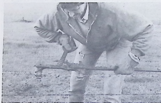
Using my trusty Red-D-Rod fence stretcher, I spliced pieces of barbed wire together. You'll notice I'm wearing gloves when handling the stretcher connected to the barbed wire. The barbs are razor sharp and even cut through the heavy cowhide gloves I was wearing.
