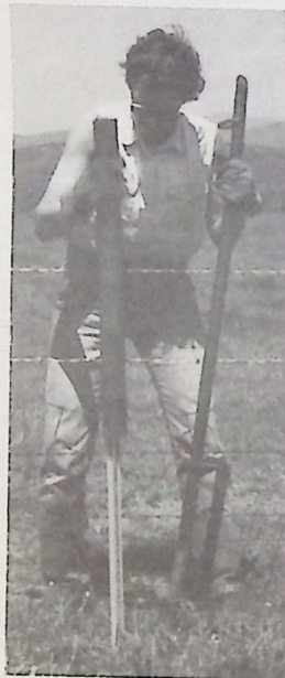
Once the wire was stretched, steel posts were driven into place.
